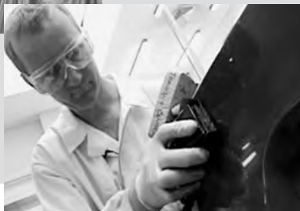
A low-energy UV lamp is used to cure the primer.
